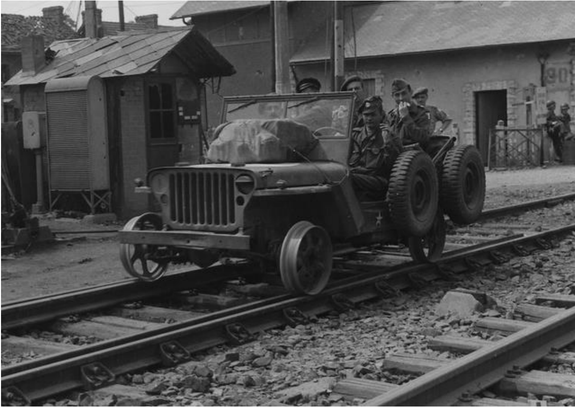
Jeep in World War II Railroad wheels on these jeeps could easily be changed into regular rubber road wheels.
